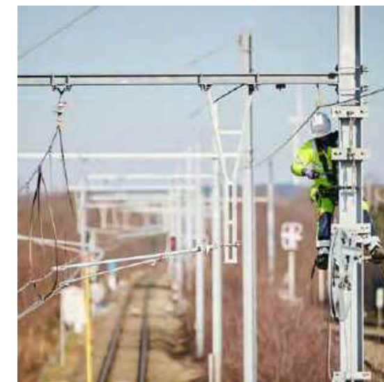
Electrification works between Genk-Goederen and Bilzen (L21C)
