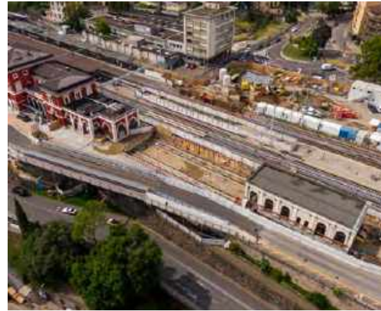
Lugano-Besso underpass construction site.
