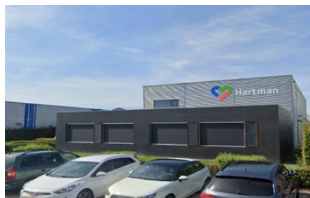
Hartman Installation - Urk
